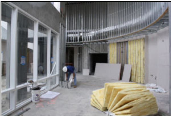
Metal Framing Defines New Lobby of Youth Center & Gym
